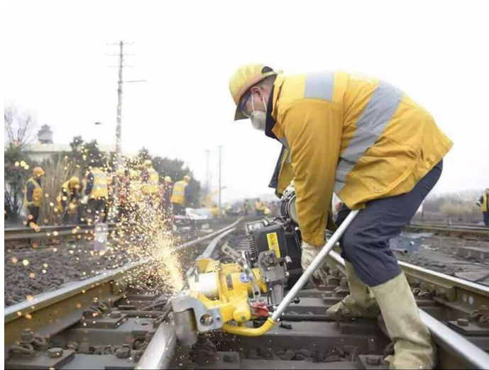
Rail Grinding
