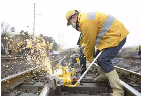
Rail Grinding
